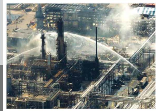
Texas City Refinery 2005
