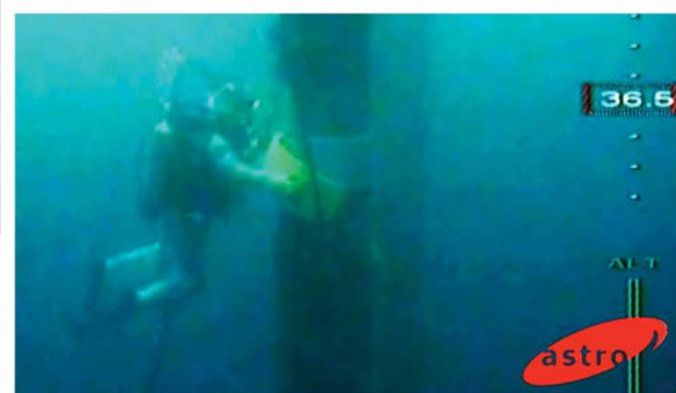
Clamp Installation
