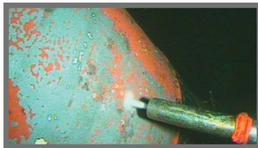
Cleaning with Water Jet
